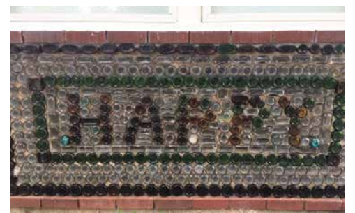
The Bottle House Museum, in Kaleva, was built using multi-colored bottles from a former bottling factory in the village. Photo by P.G. Misty Sheehan.
