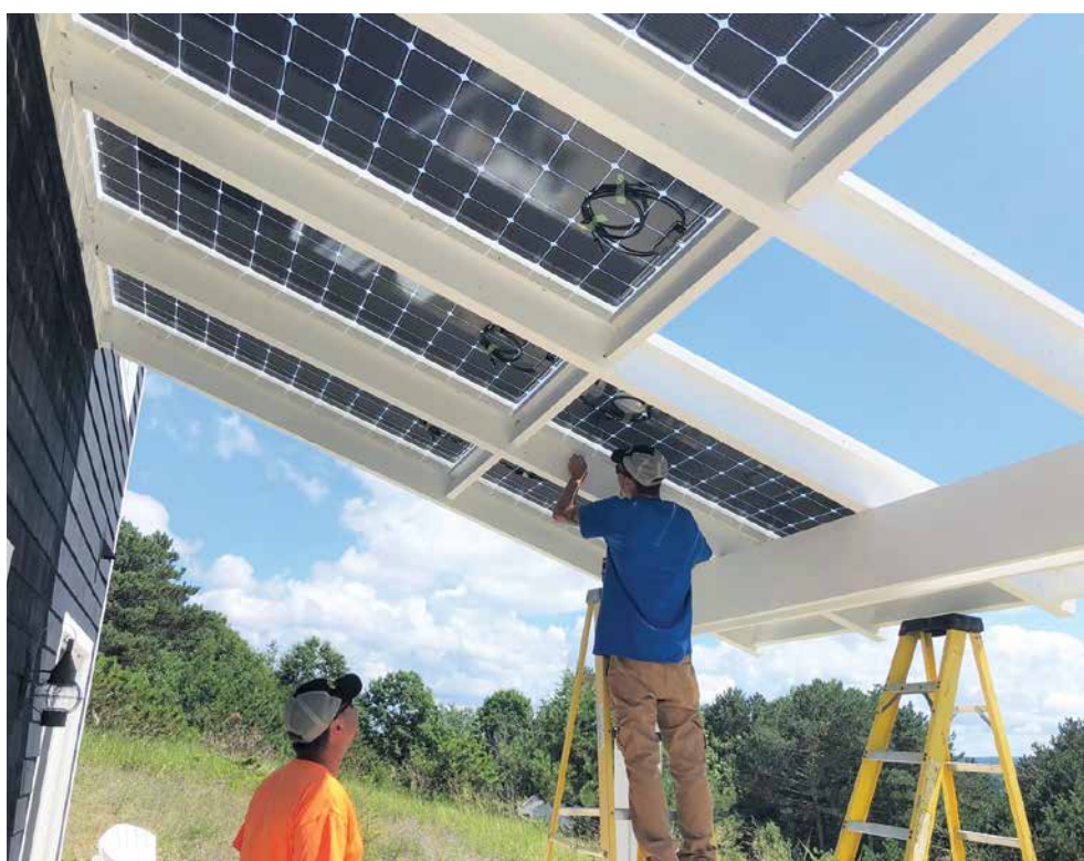
CBS Solar crew installs solar panels on a pergola. Courtesy photo
