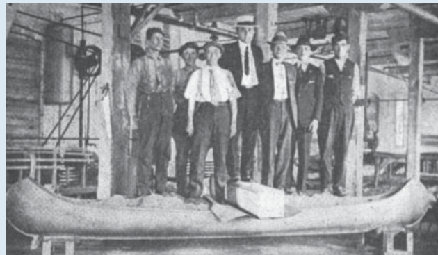
Above. Curtiss NC-4. Right. Haskell Canoe weight test. 3200 lbs. supported by a 57 lb. canoe. Henry Haskell is third from right in a bowtie. Photos in the public domain.
