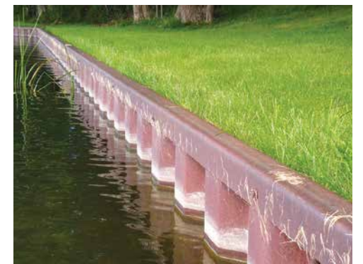
Armored lakefront. Photo by S.A. McFerran.
