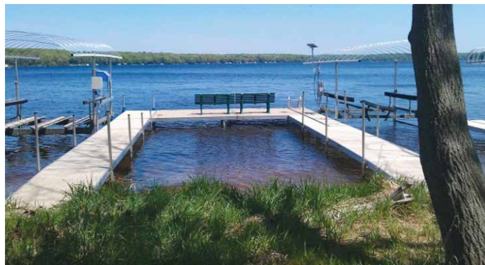
Carie's Marine & Home Construction, of Ludington, installed this flow-thru dock with dual boat lifts. Courtesy photo.
