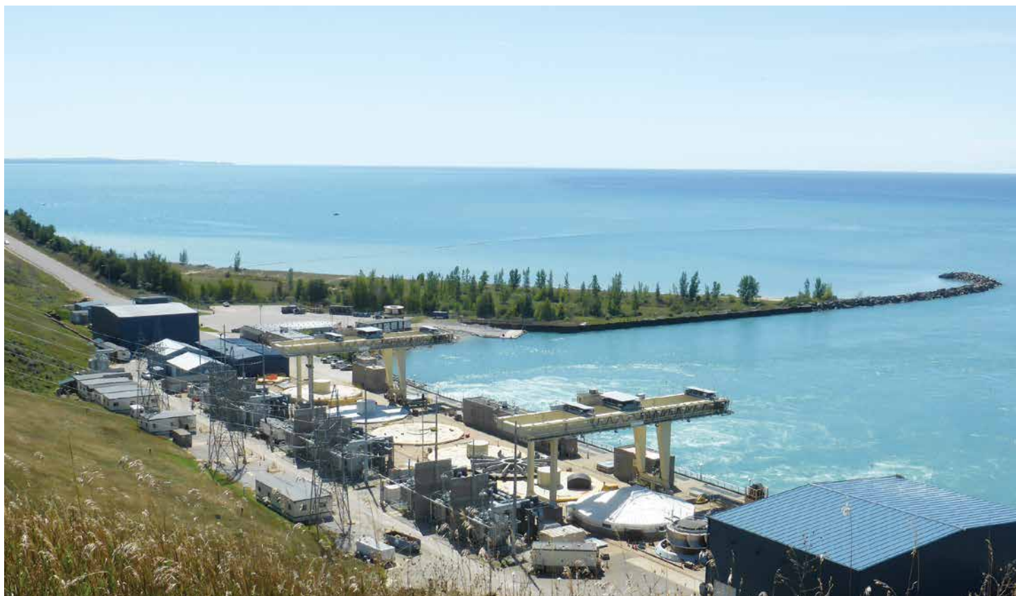
The view from the overlook at Ludington Pumped Storage provides a wide vista of Lake Michigan, with the facility below. Photo by Mark Videan.
