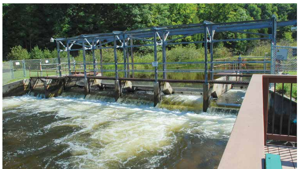
The weir at Little Manistee River. Photo by Kevin Howell.
