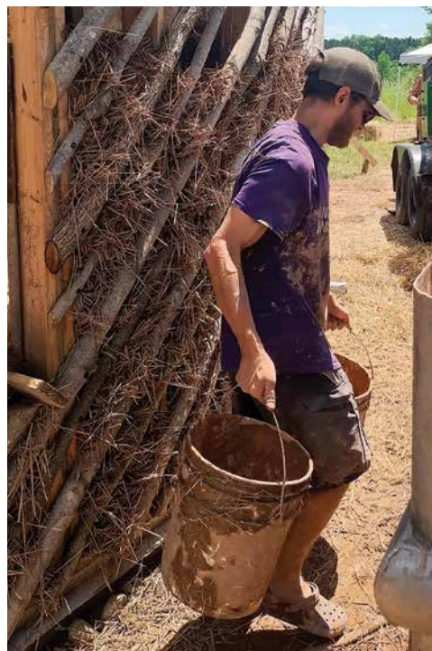
Todd Gerardot is part of the mud-mixing team.
