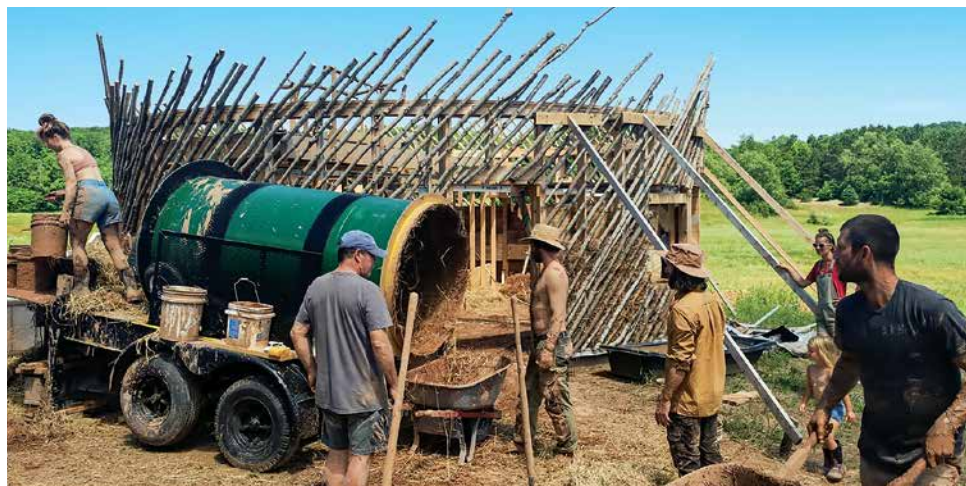
The drum mixes clay and straw.
